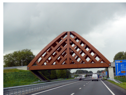
Bridge in the Netherlands from acetylated pine WOOD. Photo: Gerhard Büttner, CC BY-SA 3.0.
