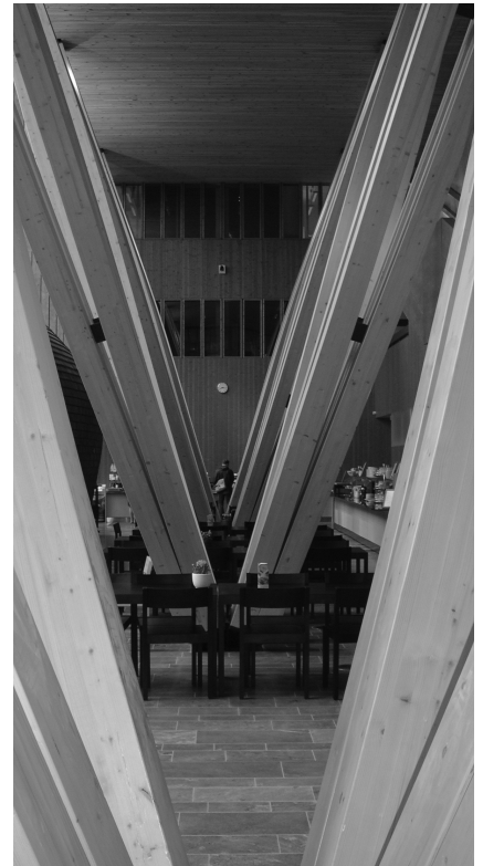
The Metla building in Joensuu is an example of the increasing interest in wood technology. 2000 m 3 of wood was used in its construction, in many innovative ways.
